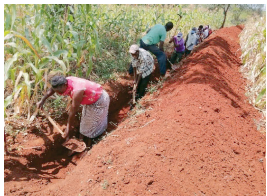
Members from different groups establishing soil and water conservation structures through communal work
