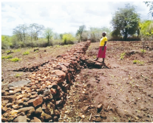
Use of stone lines & interrupted terraces
